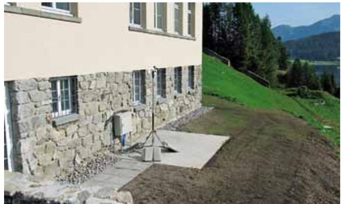
Figure 5. Foundation for the Heliostat at the south-east face of the institute building.
